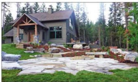
Lowe helped to restore a home that was flooded by a lake that rose above the official high water mark. The home was physically picked up and moved, and the grounds restored better than they were with Lowe's touch. (Courtesy of Leslie Lowe)
